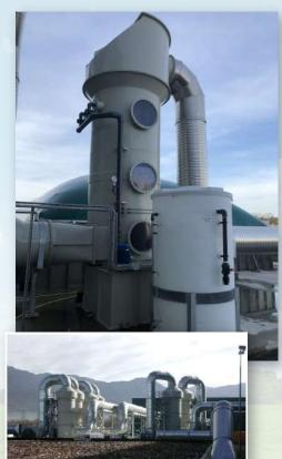
Scrubbers can operate as a single-stage or multistage systems; in this latter case, different chemicals are sequentially used for pollutants removal (for instance, first stage: sulphuric acid; second stage: sodium hydroxide). Other configurations (i.e., horizontal fixed-bed scrubber, co-current or cross-flow configurations) can be realized.
